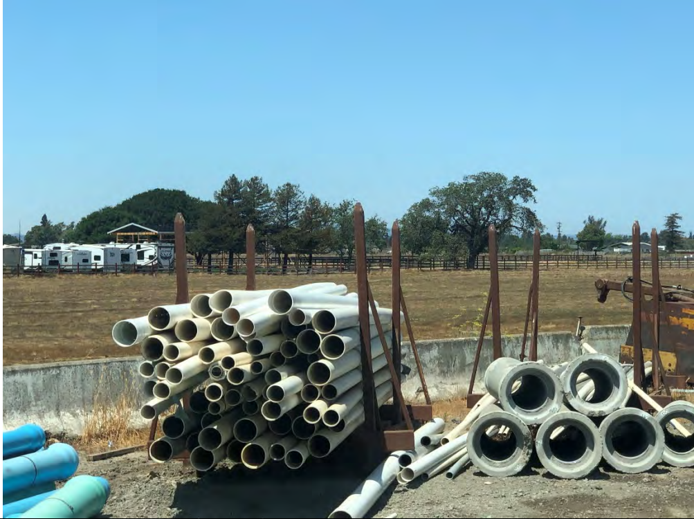
Concrete k-rail prevents CTS from dispersing into stockpile and staging areas on the site.
