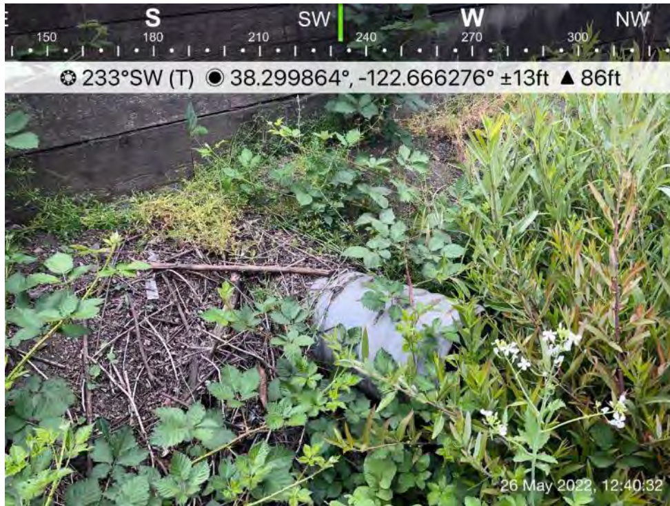
Photograph 7. View of CMP that runs beneath Adobe Road in the northeast corner of intersection that outfalls into unnamed intermittent drainage (ID-01).
