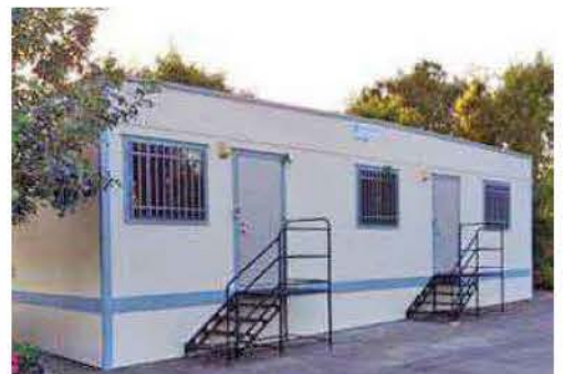
OFFICE TRAILER EXAMPLE
