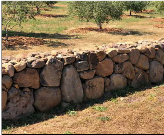
DRY STACK LOCAL STONE WALLS
