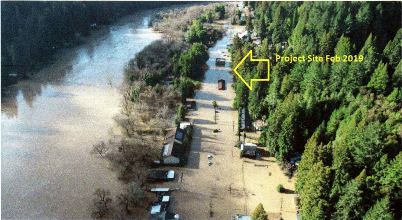
Feb 2019, water over dispensers and to near the roof of brown roofed building in previous photo
