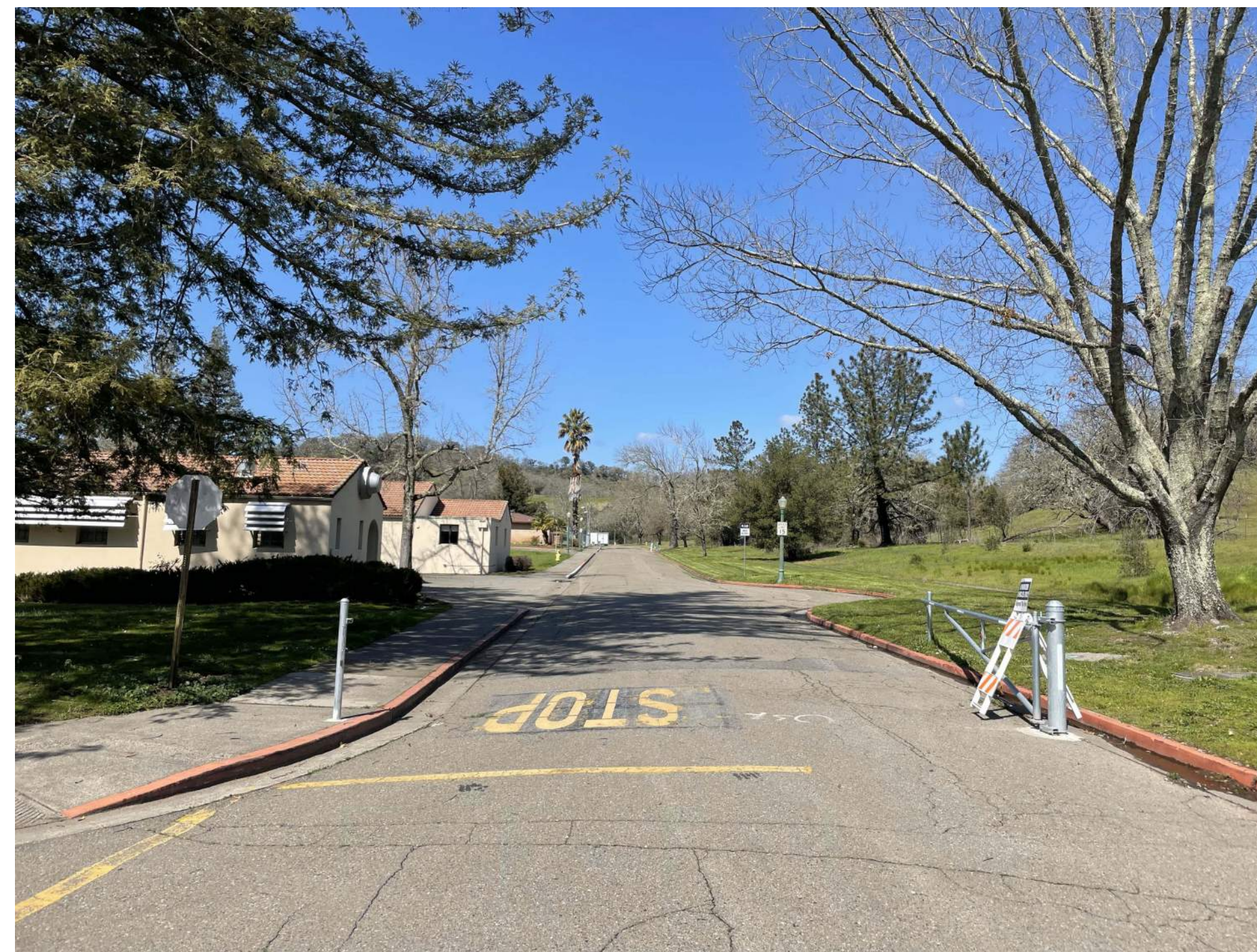
Looking North down Railroad Rd
