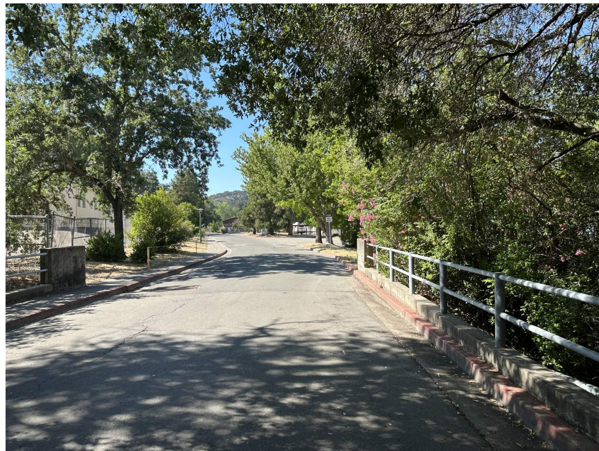
Looking north across the Sonoma Cir. bridge
