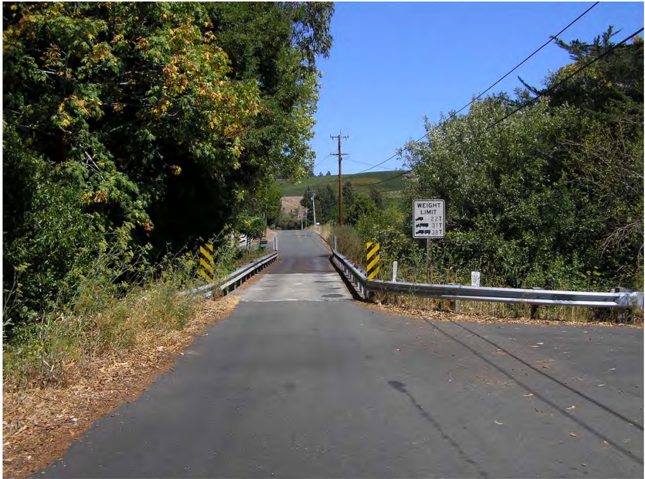
Figure 8 View of Freestone Flat Road Looking Northeast
