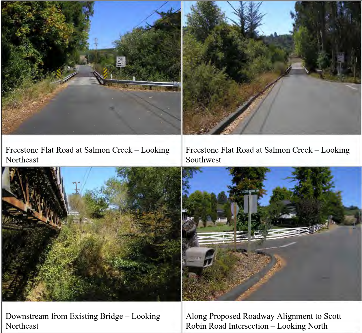
Figure 4 Project Site Photographs
