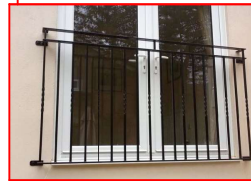
JULIET RAILING AND DECK RAILING PAINTED, HOT DIPPED GALVANIZED STEEL OR SIM.
