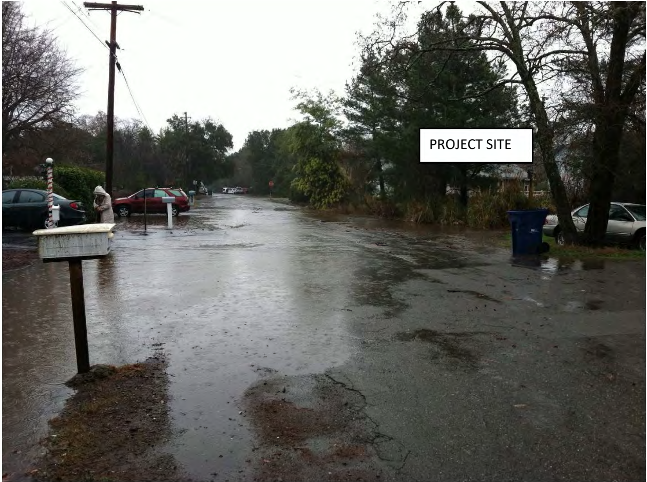
Figure 4 - Walnut Avenue looking east from Linden Street (viewing excess flood flows from Linden Street now flowing east on Walnut and overtopping Walnut Avenue toward proposed project site).
