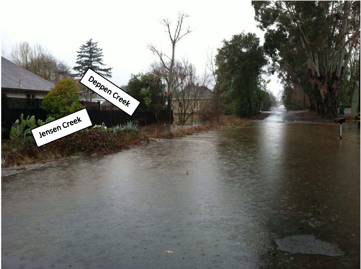
Figure 1 - Linden Street looking north from Walnut Avenue (viewing road overtopping at confluence of Deppen Creek with Jensen Creek)
