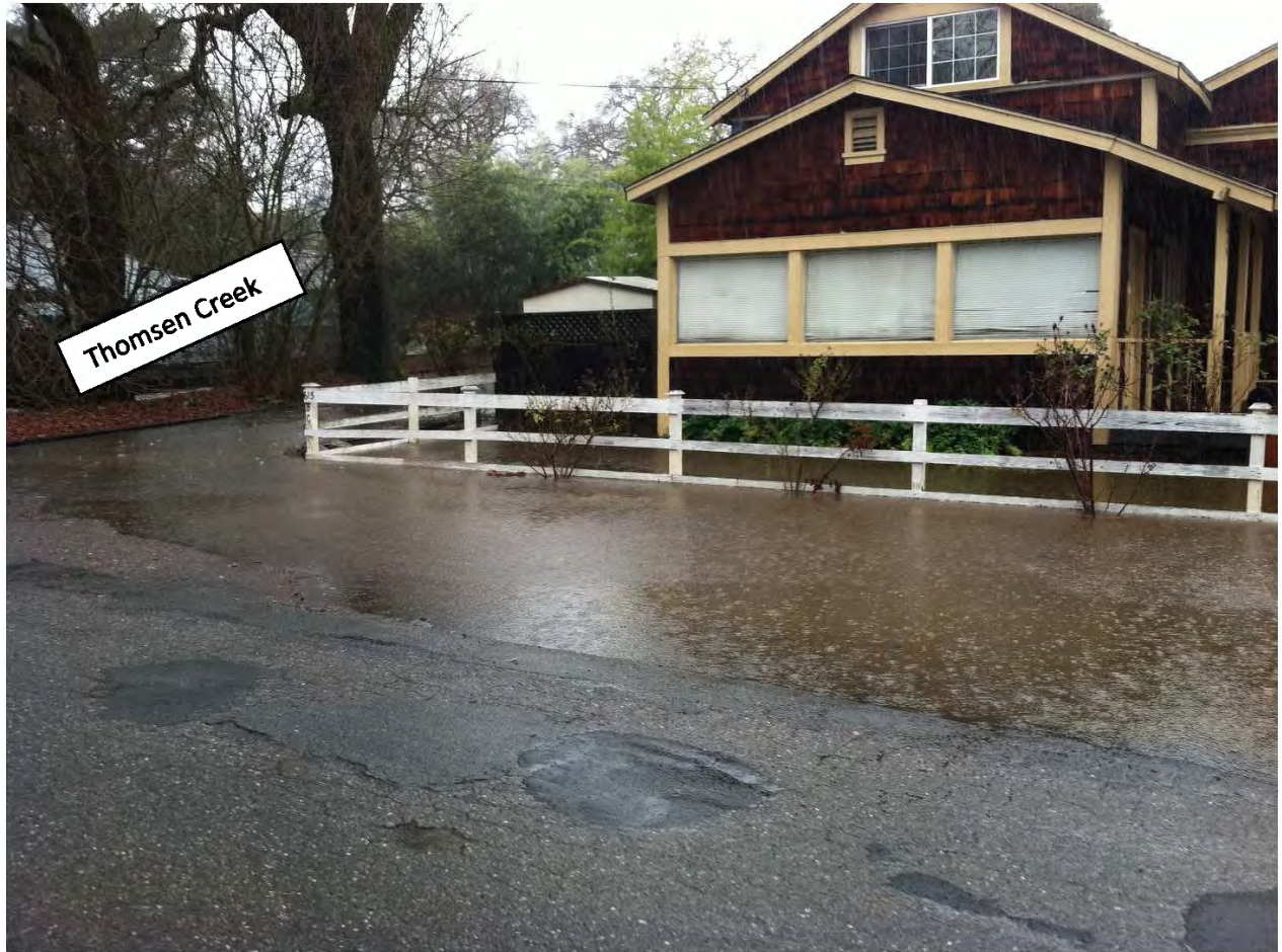
Figure 7 - Overland flood flows from project site remain overland along Thomsen Creek corridor downstream of project site (viewing same parcel as Figure 6).
