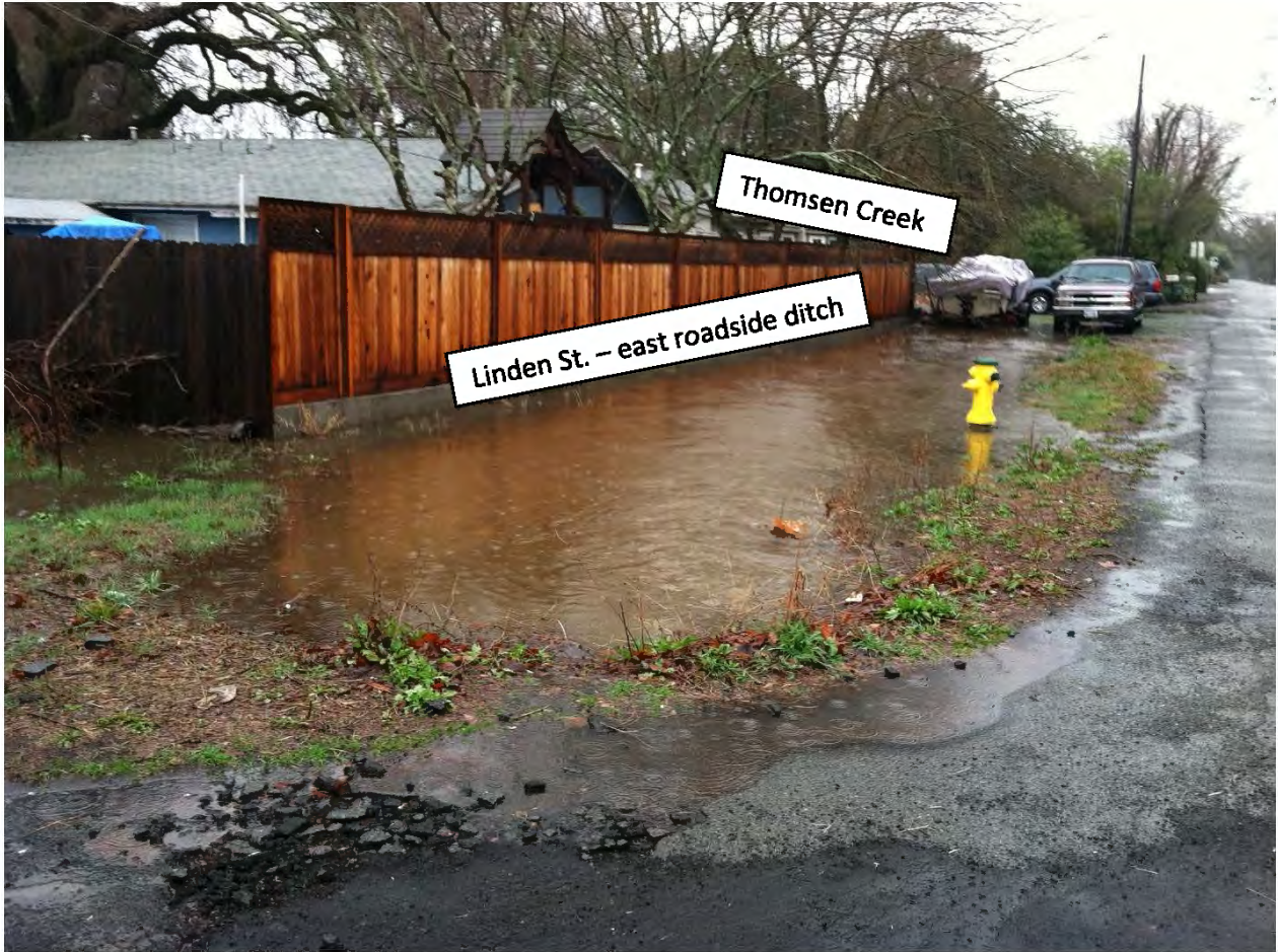
Figure 3 – Linden Street looking south from Walnut Avenue (viewing east roadside ditch back-watered from Thomsen Creek confluence)
