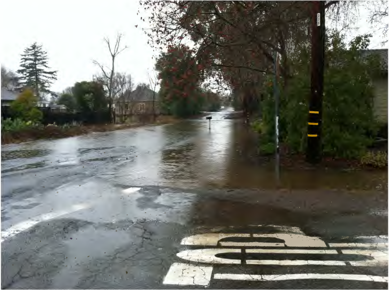
Figure 2 - Linden Street looking north from Walnut Avenue (viewing east roadside ditch becoming overwhelmed from Jensen Creek overtopping Linden Street)
