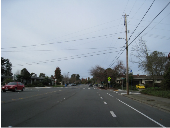
FIGURE 3.1-4 EXAMPLES OF EXISTING ROADWAYS WITHIN THE PROJECT AREA
