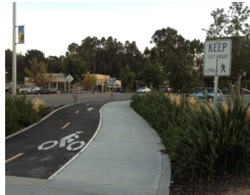
Coffey lane extension pedestrian/bicycle path
