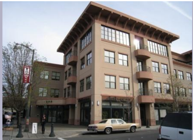
Offices over retail/service
