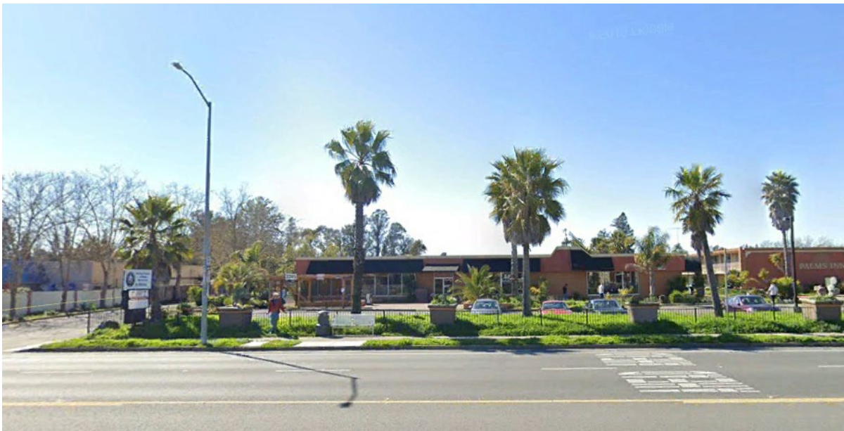
Figure 4.1-31 SAN-4 from Santa Rosa Avenue, Looking West
