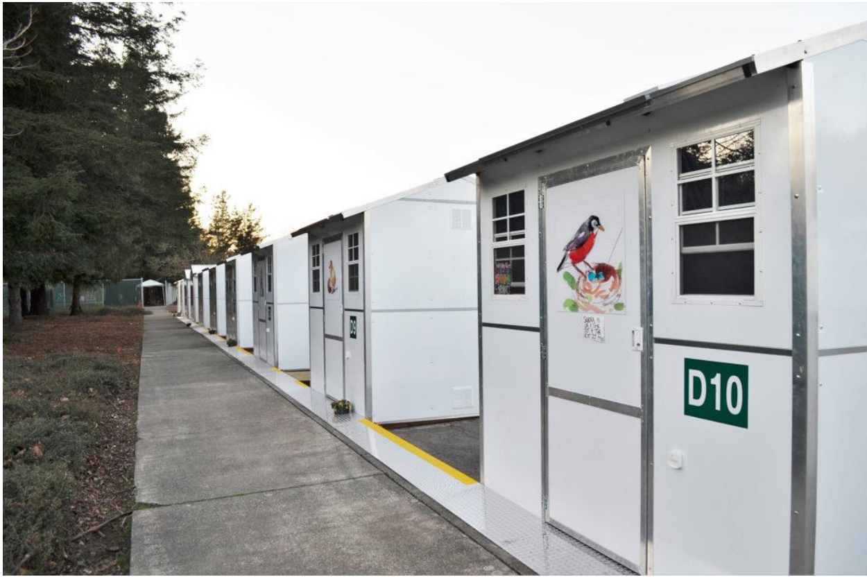
Figure 5: Los Guilicos Transitional Shelter Units
