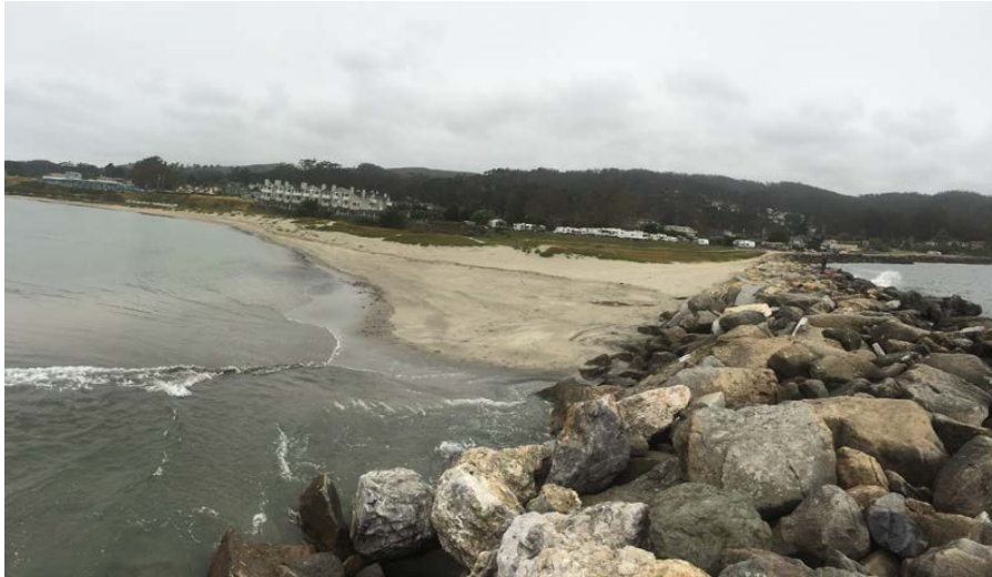
Figure 4.10. Panoramic view taken from the east breakwater looking east at the sand shoal accumulated inside the harbor (left side of groin). (Photo: Max Delaney)
