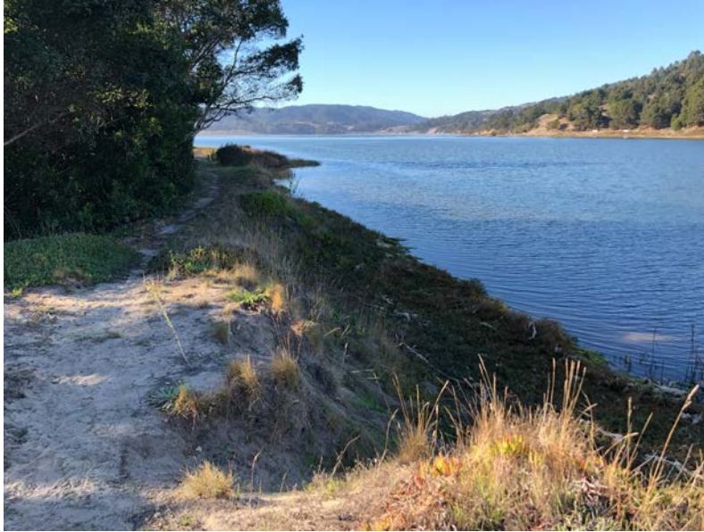
Figure 4.7. Eroded section of shoreline and steep ~10-foot scarp along Dipsea Road. An unmaintained recreational trail that runs for most of the length of Dipsea Road is located within the vegetated area along the shoreline. Erosion threatens the stability and accessibility of the trail. (Photo: Wendy Kordesch)
