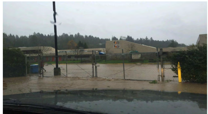
Water rushing down Marys Ln & into school
