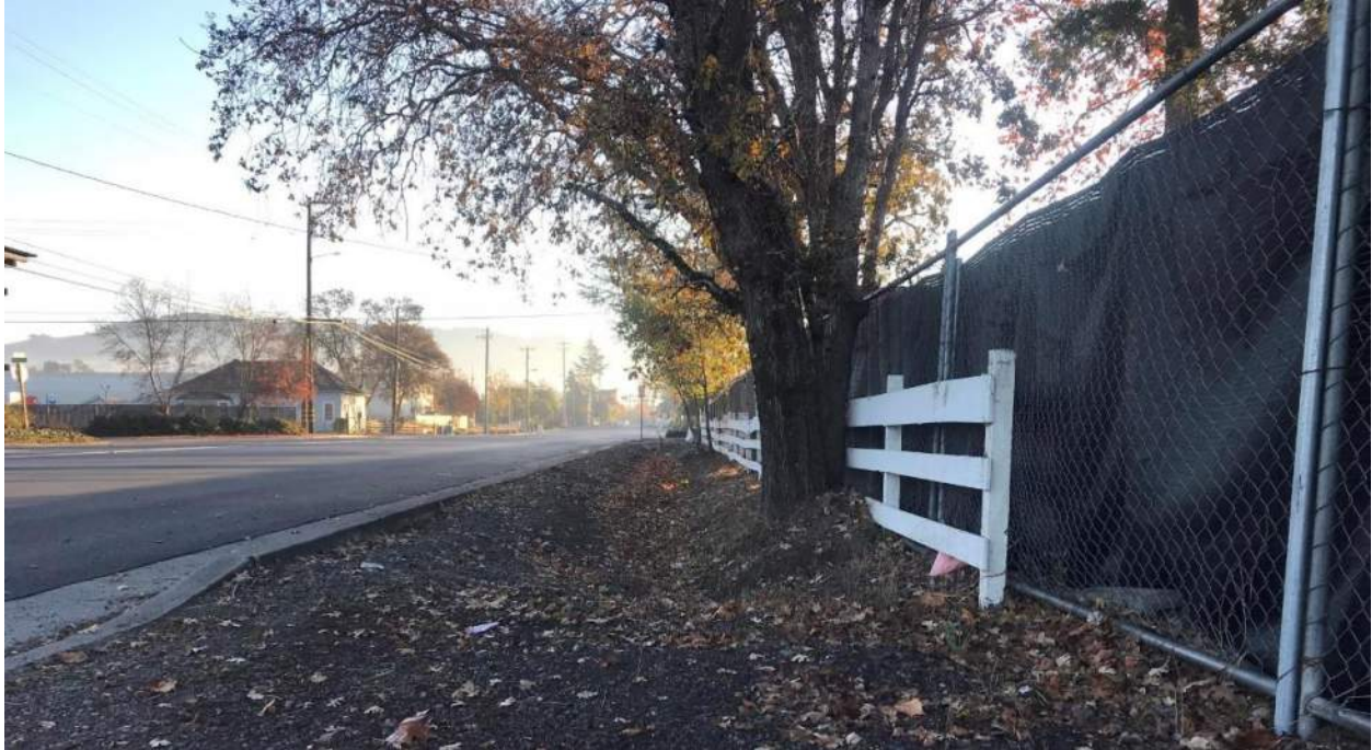
Photograph 15. View of drainage ditch on south side of Todd Road, from west end of easternmost segment, facing east.
