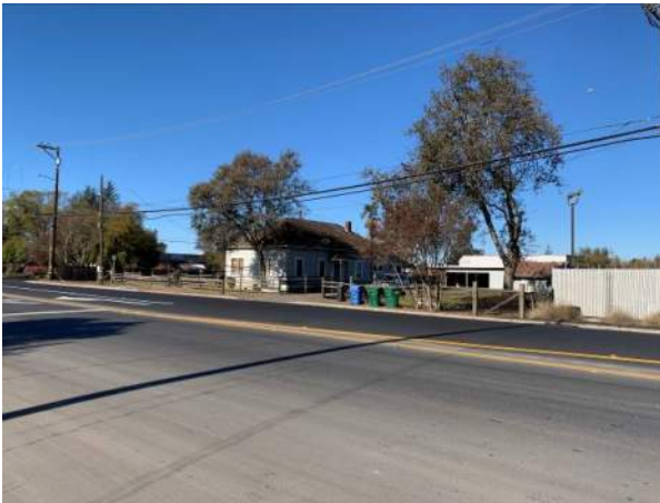
Photograph 4. View of abandoned home on the west end of the subject property.
