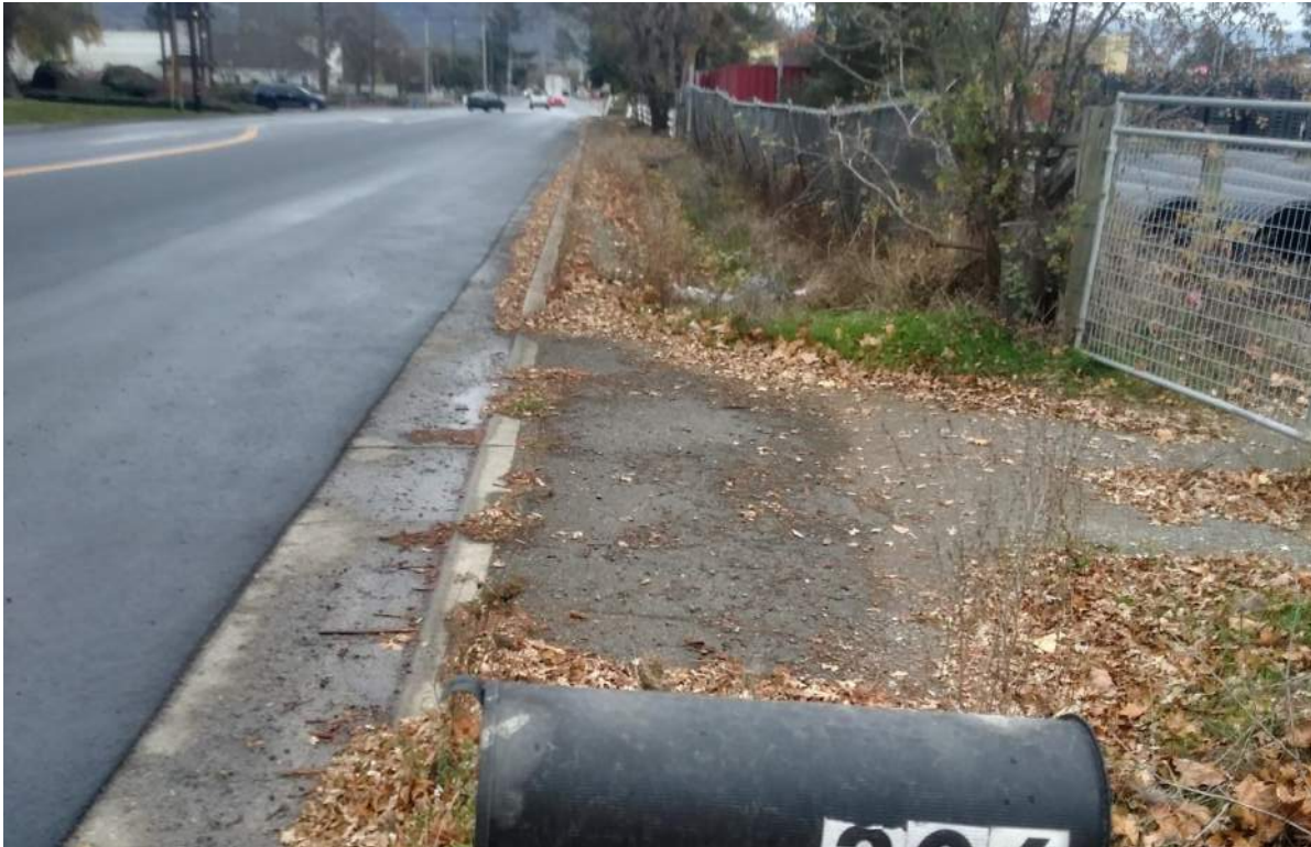
Figure 5 View of Western Portion of Project Site - South Side of Todd Road, Slightly West of Standish Avenue, Looking East
