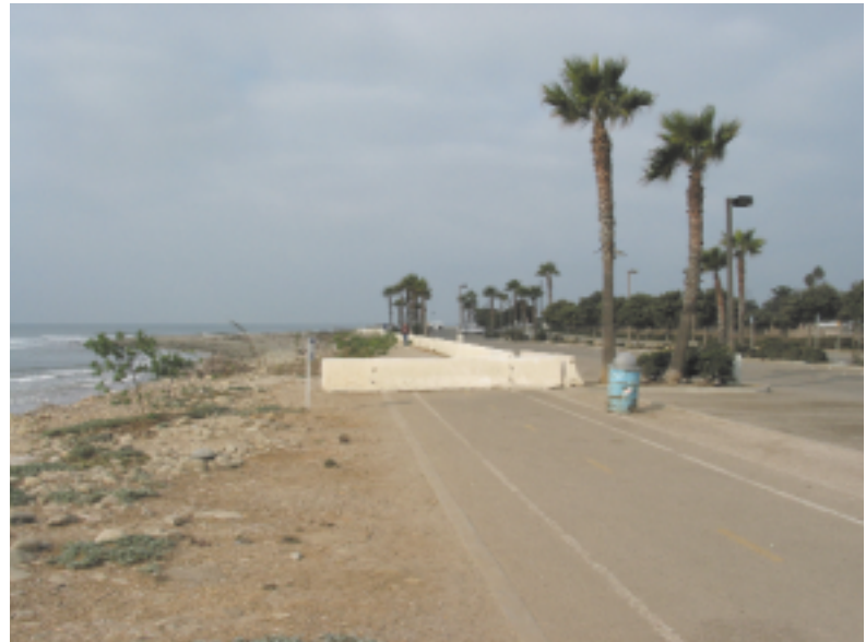
Eroded shoreline at Surfer's Point, Ventura County
