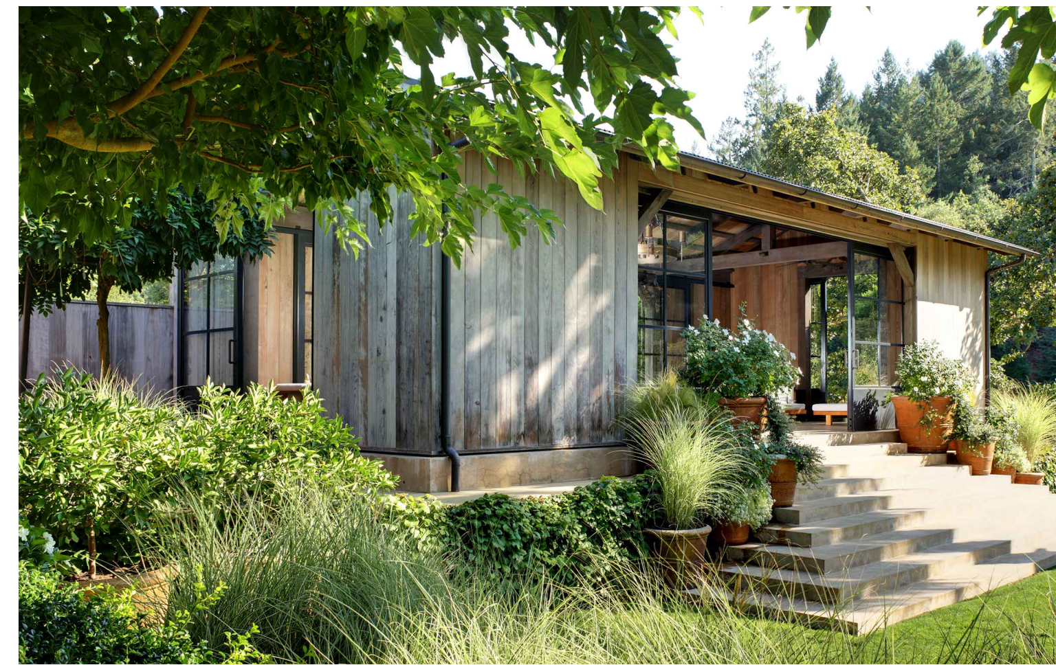
VERTICAL BUTT JOINTED SIDING
