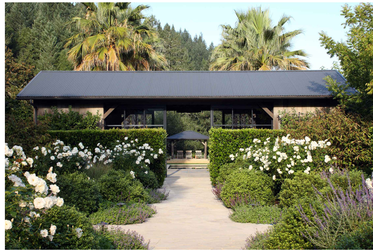
CORRUGATED METAL ROOF
