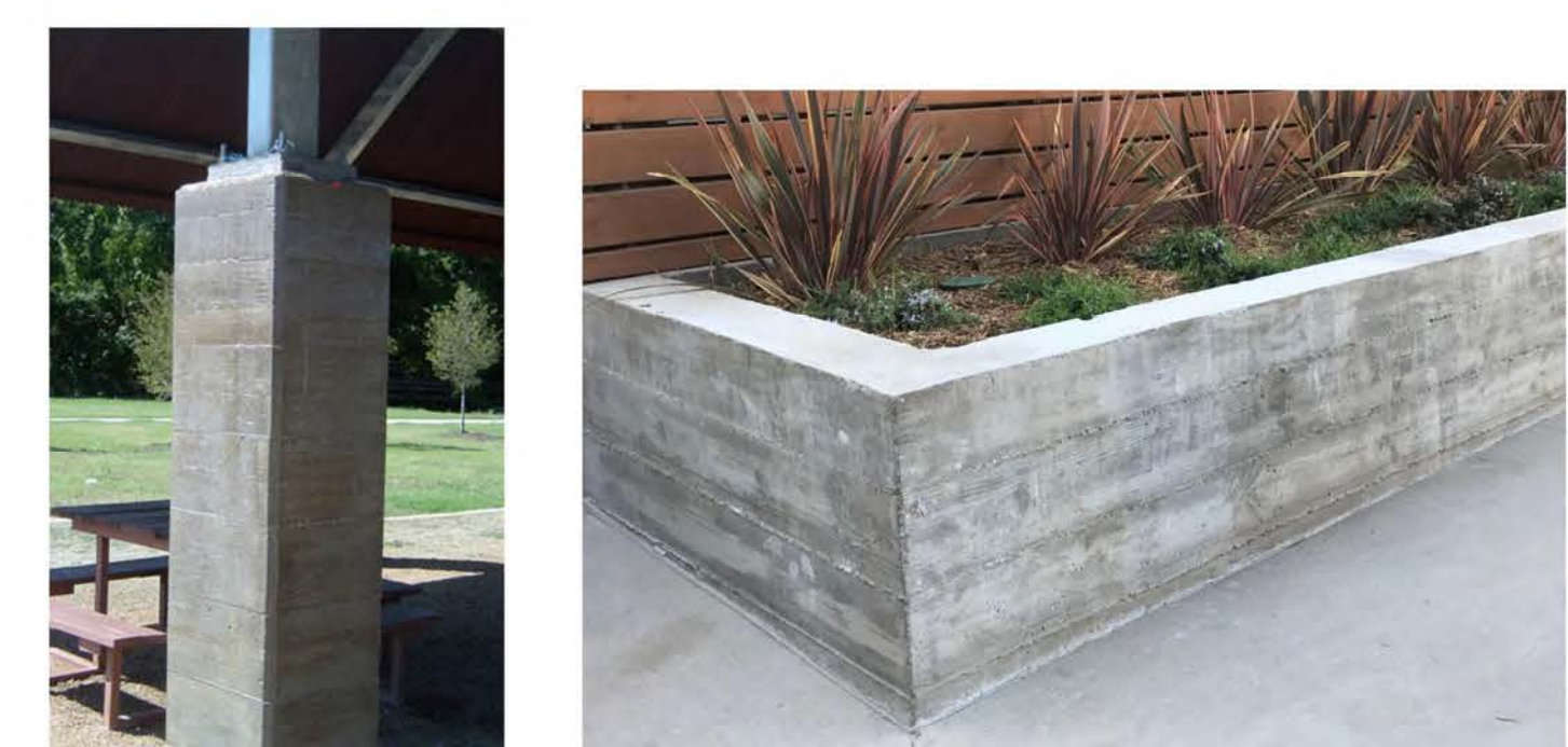
3 BOARD FORMED CONCRETE IMAGES 1/2" = 1'-0"
