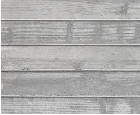
WALL 01: CONCRETE FOUNDATION > Board-formed
