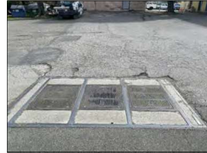
EXISTING PG&E S.S TRANSFORMER T-8279 VAULT
