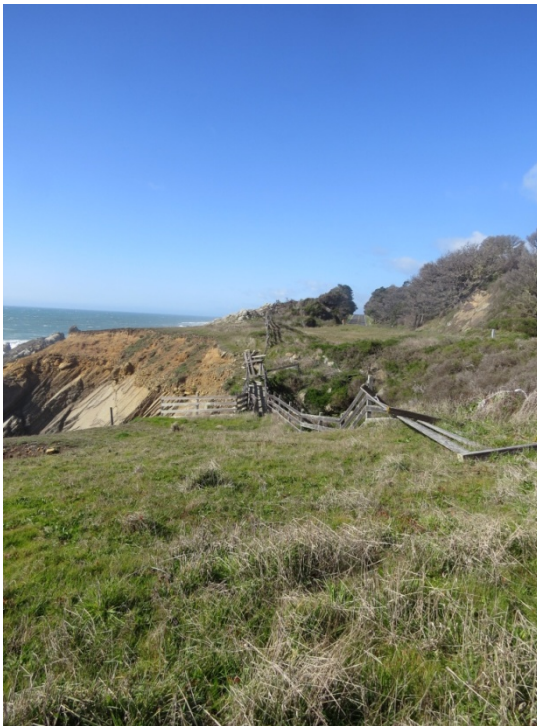
Photo 1 - Historic Wooden Bridge
