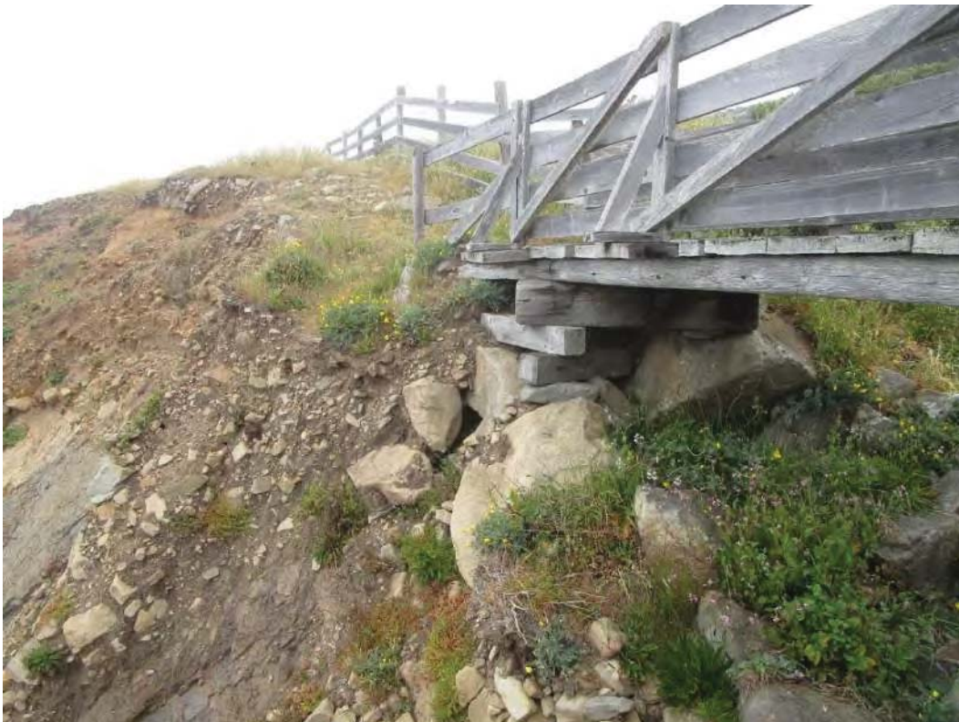
BRIDGE 2 NORTH ABUTMENT, LOOKING NORTH
