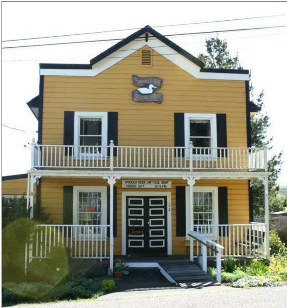
Figure 14 - False front on former Druid's Hall
