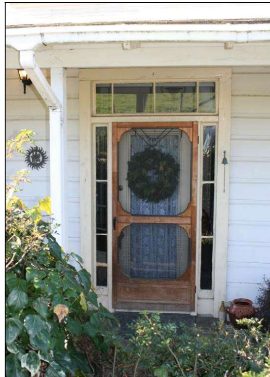
Figure 21 – Screen doors and transom windows allow air circulation
