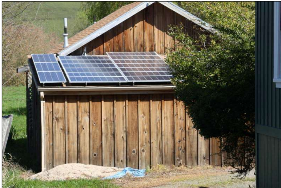
Figure 22 - Solar panels discretely placed on an accessory structure
