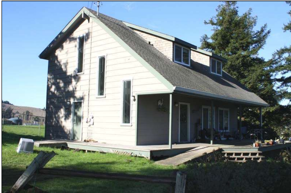
39 – 17123 Bodega Lane, APN 103-120-026
