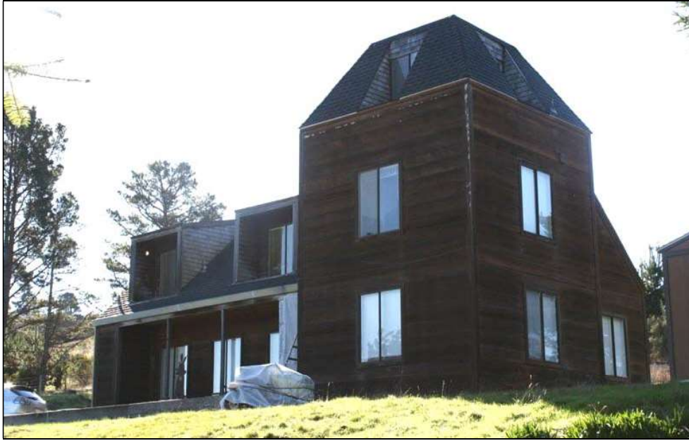
44 – 17500 Bodega Lane, APN 103-010-034
