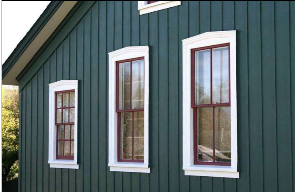
Figure 11 - Double-hung windows in Bodega Historic District
