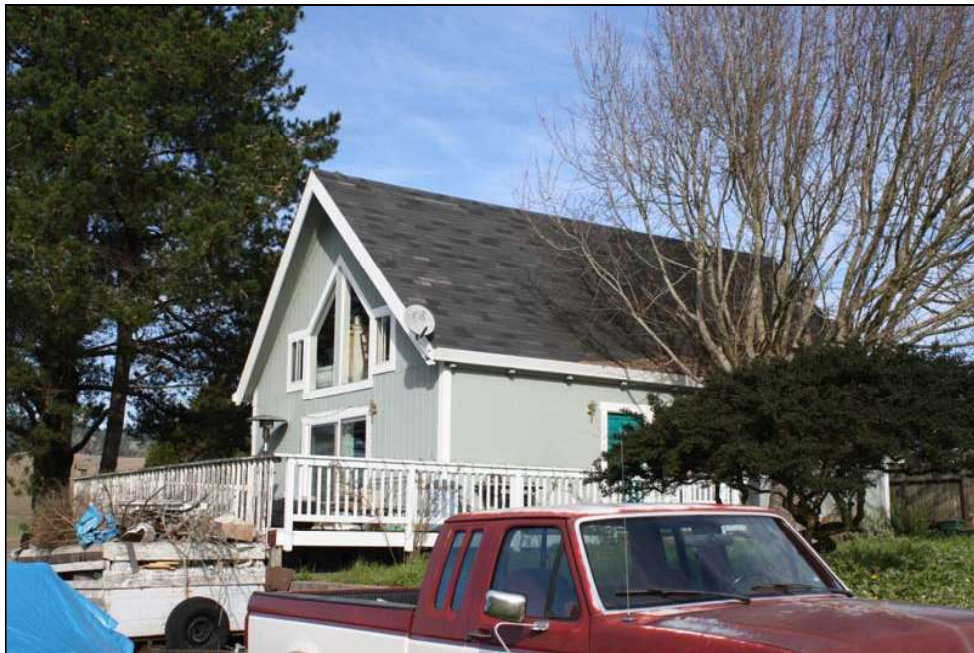
43 – 17299 Bodega Lane, APN 103-120-017
