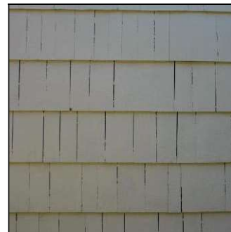
Coursed shingle siding
